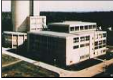
AVR, Germany 15 MWe 1967-88
