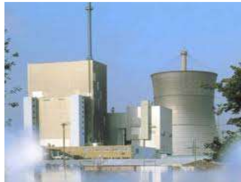
THTR, Germany 300 MWe 1986-89
