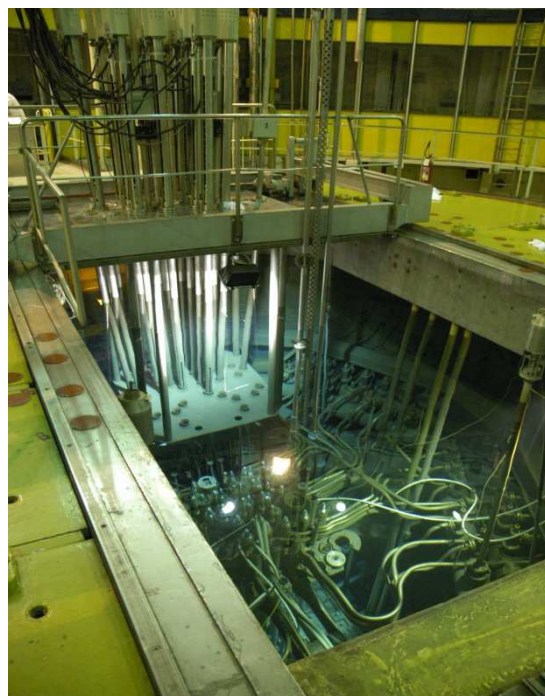
Fig. 2. View of the reactor pool.
